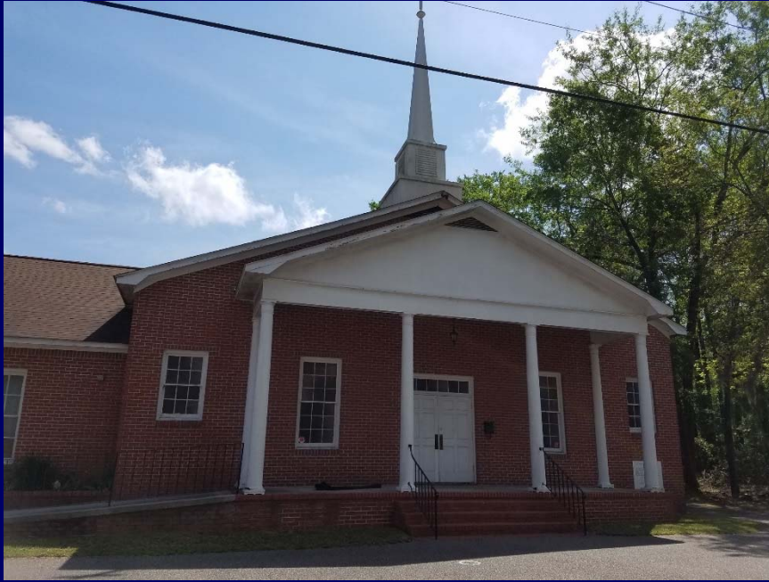
3 – Adjacent Property (Church on Main Rd)
