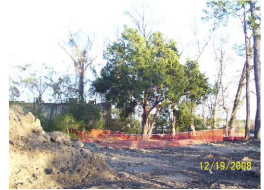
Tree Protection Fencing
