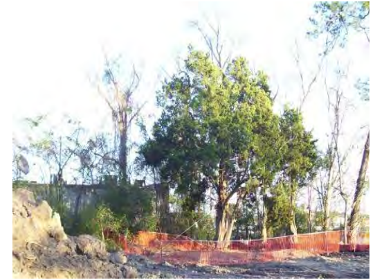
Tree Protection Fencing
