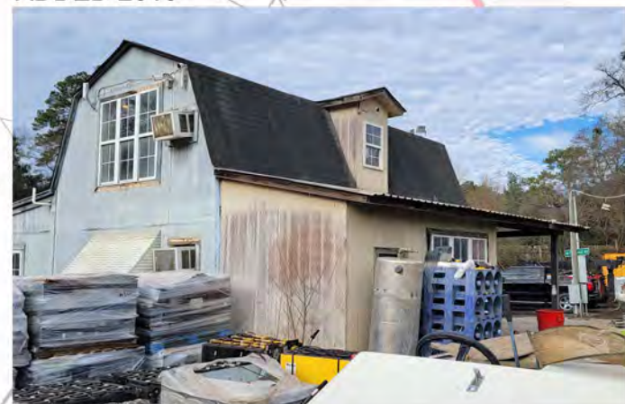
ORIGINAL OFFICE BUILDING EXTENSION - ADDED 2010
