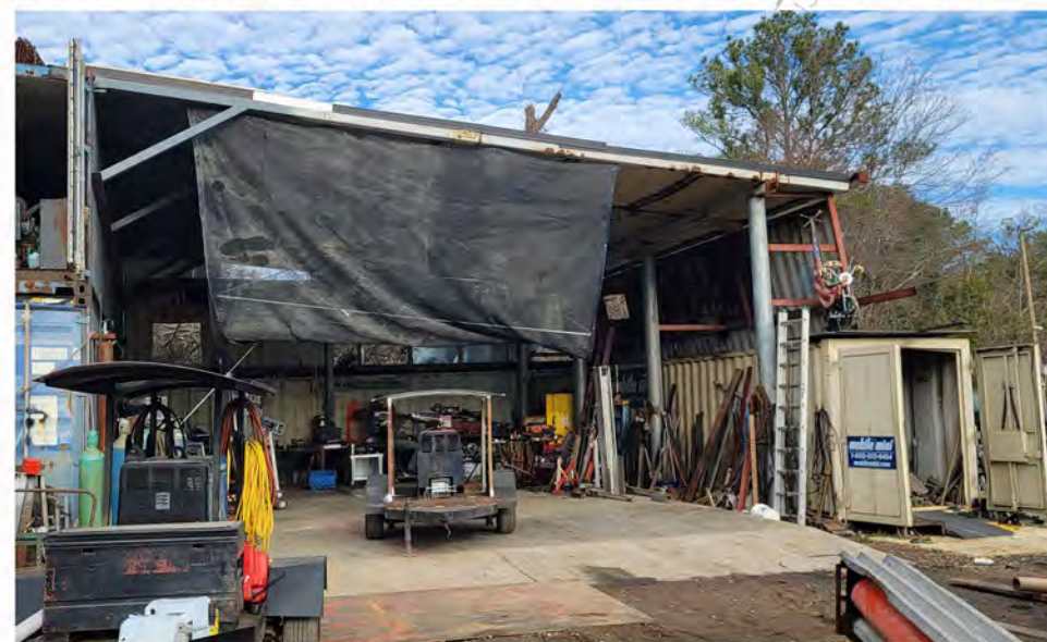
METAL SHED ADDITION TO CONTAINER SHED - ADDED 2019
