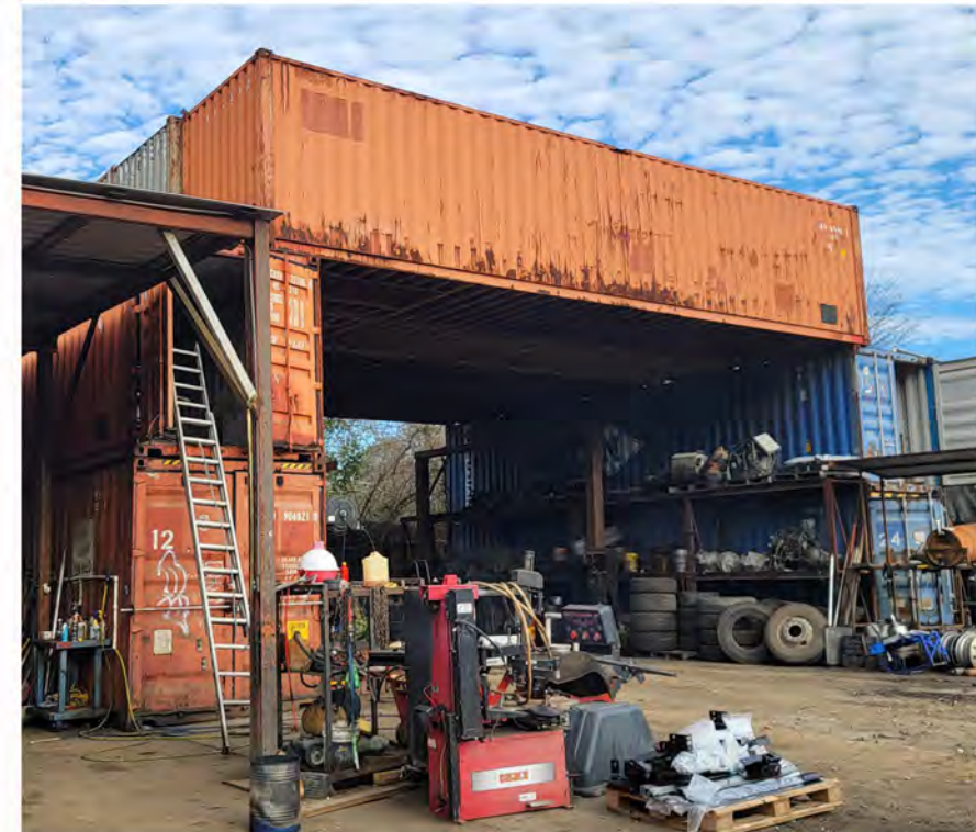
CONTAINED SHED REPLACING ORIGINAL SHED - ADDED 2014
