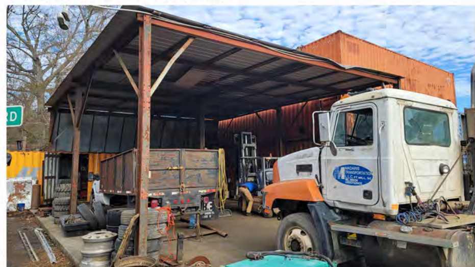
ROOFED AREA - ADDED 2011
