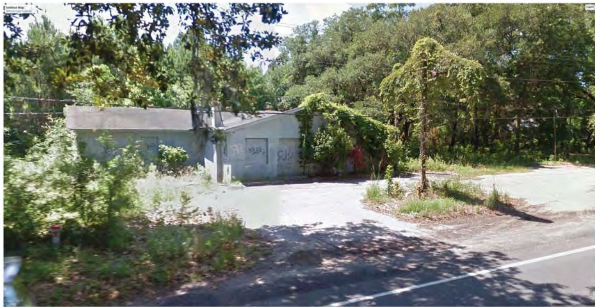
EXISTING CONDITIONS ON SITE - ABANDONED BUILDING, OVERGROWN VEGETATION, ETC.
