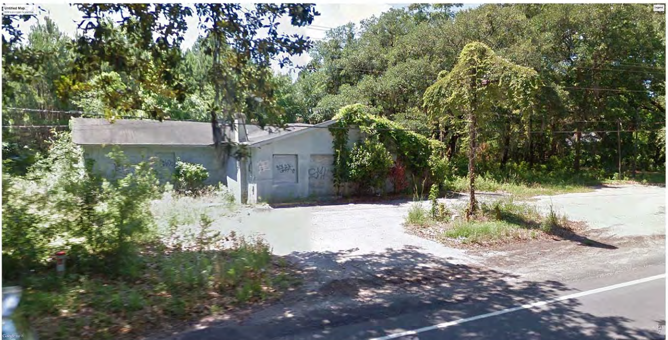
EXISTING ISLAND GROCERY ON PARCEL
